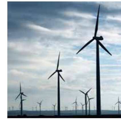
Energy Management System according to ISO 50.001
