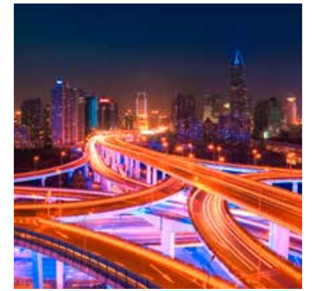
Intelligent Traffic Control System
